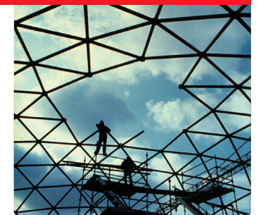
La Géode nears completion. This Buckminster Fulleresque dome, built in Paris in 1985, uses 1,670 steel triangles.
